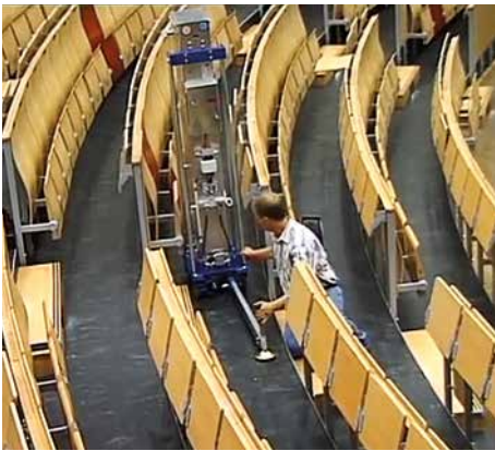
Fitting of the lower outriggers
