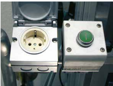
Power supply in the work cage
